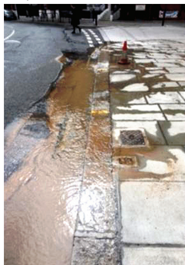
Flooding outside the church caused by burst water main...
